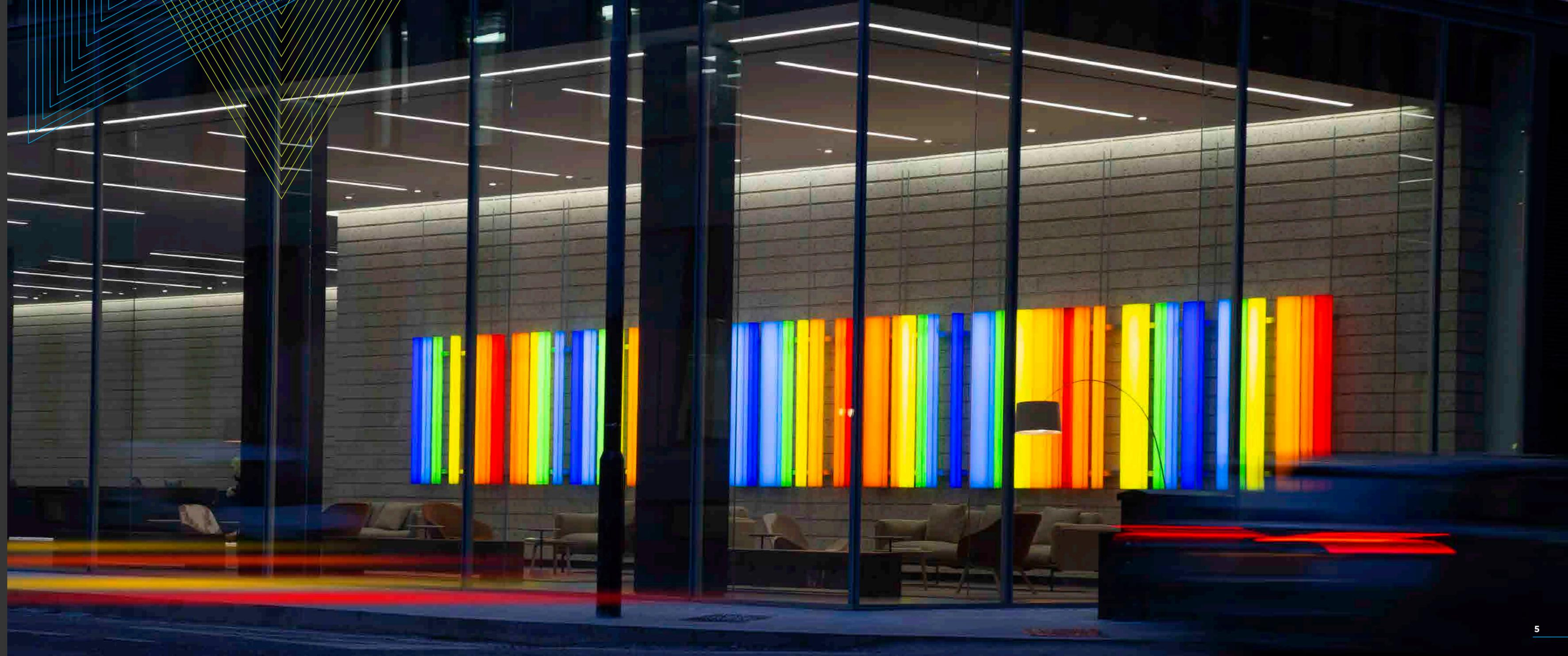
**THE TECHNICAL DETAIL:** This unique installation comprised a series of vertical neon lighting panels that spelt out the building name, One Bartholomew, in barcode. The complex cabling for each panel was designed to sit within a narrow MF ceiling detail inside a series of recessed lighting troughs that were set in front of a mechanically fixed stone wall cladding system.
